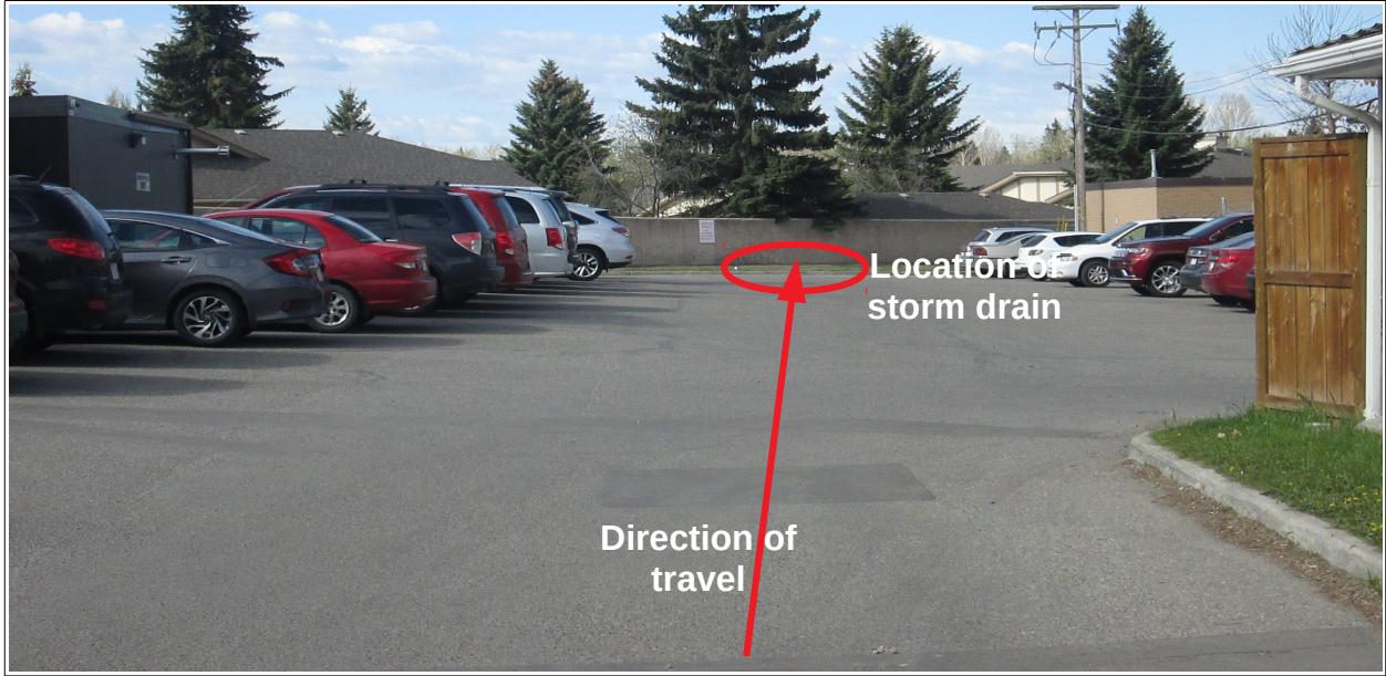
Figure 6: View of Segment 2 route through a parking lot.
